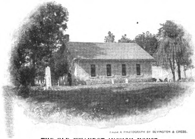
FROM A PHOTOGRAPH BY BELVINGTON & CRESS. THE OLD WYANDOT MISSION HOUSE.
