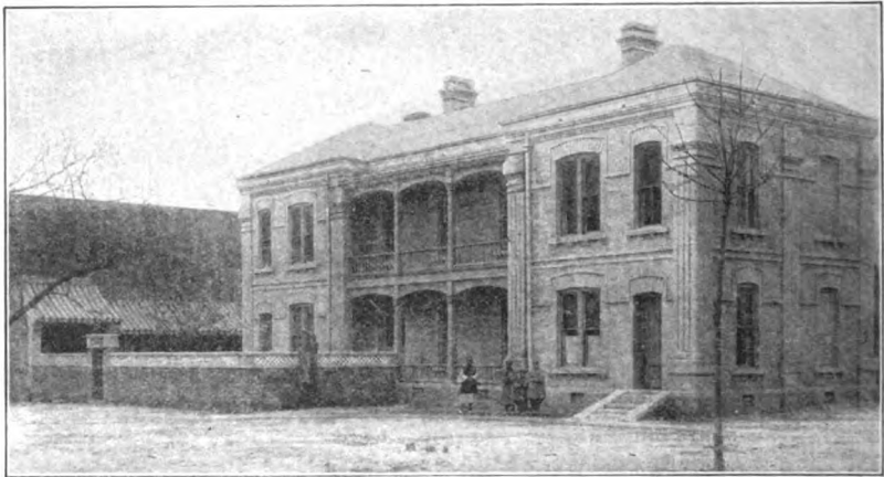
SLEEPER DAVIS MEMORIAL HOSPITAL, PEKING.
