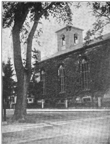
OLD SOUTH CHURCH, PORTSMOUTH.
